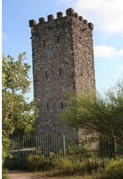
Stone tower at Comanche Lookout.
